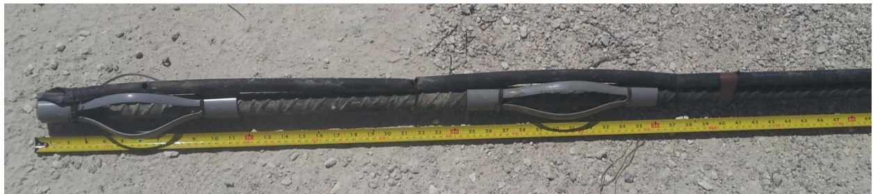
Figure 23 - Detail of the lower part of each anchor, as assembled prior to insertion.
