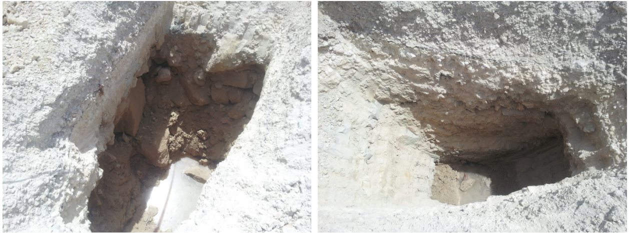
Figure 30 - two of the trial pits excavated during this investigation
