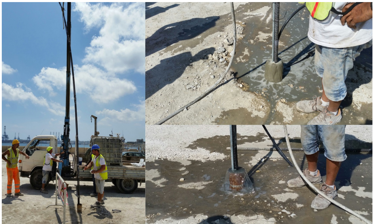
Figure 24 - Details of the pull-out test anchors construction process
